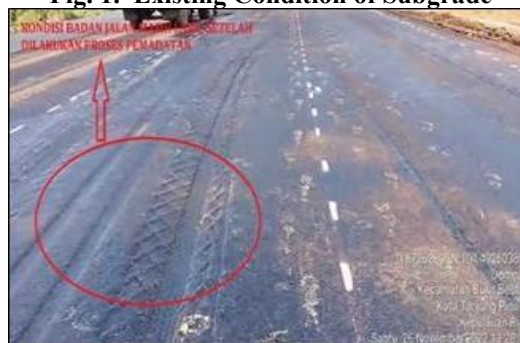
Fig 2. Subgrade remains soft after compaction [2]
