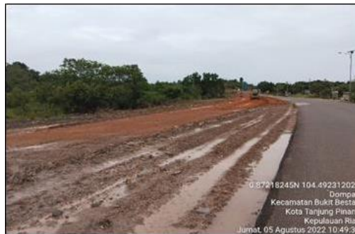
Fig. 1. Existing Condition of Subgrade
