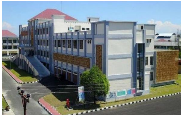
Fig. 1. Integrated Laboratory Building of Padang State University
